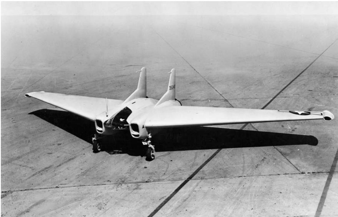
John K. ("Jack") Northrop designed numerous advanced aircraft of conventional configuration, but he was fascinated by the flying-wing concept. He believed that such a pure airfoil surface would have the most efficient lifting capabilities. Also, the absence of a fuselage and tail unit would mean less drag to affect overall performance--as well as lower production costs. Shortly after designing Lockheed's famed Vega series of
